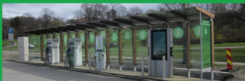
At all stations more points can be added if demand increases. One of the stations is prepared for the new generation of super quick DC chargers of more than 150 kW and can easily be upgraded as soon as the new protocols are approved.
