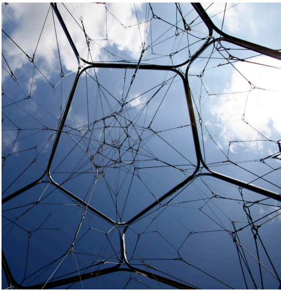
Detail of Interior Net Material: stainless steel cable of different thickness
