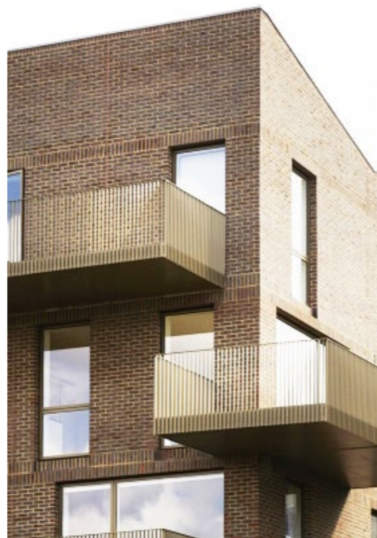
9. Räcken, takfot. Brentford Lock West, Duggan Morris Architects
