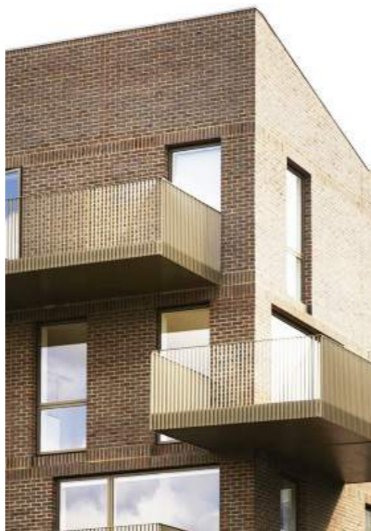
11. RÄCKEN, TAKFOT BRENTFORD LOCK WEST, DUGGAN MORRIS ARCHITECTS
