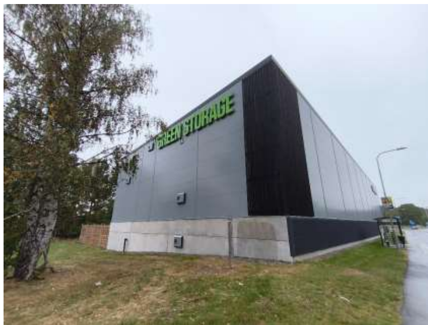
Figur 3. Green Storage lagerlokal
