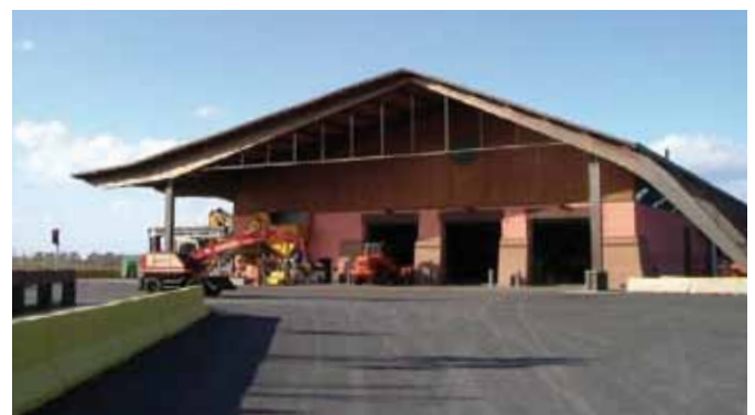
Waste Organic Treatment Plant in Maccarese
