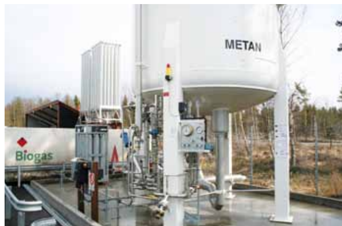
Filling of liquefied natural gas (LNG) to swap-bodies
