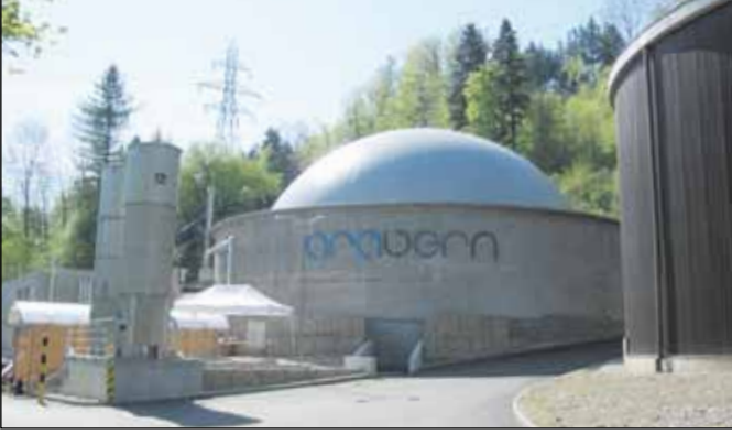
Gas storage (ballon)
