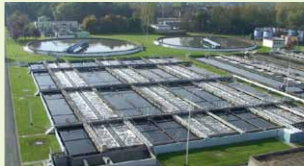
Sludge decant in bassin
