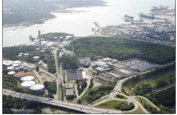
Gryaab wastewater treatment plant
