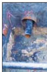
Grid and pipe before connection (Lille)
