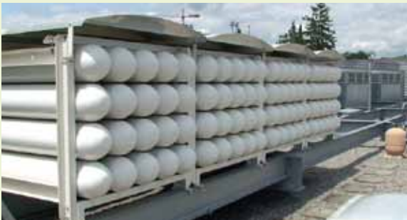
Storage facilities above the bus depot of Bernmobil
