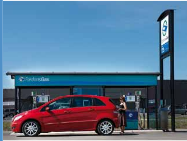
Filling station in Western region of Sweden
